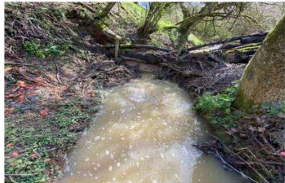
Dam silted up at the base: now acting like a debris dam
