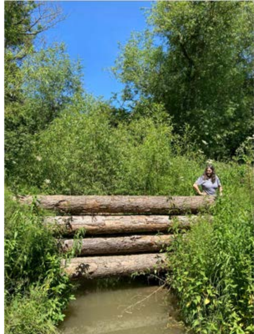
New style leaky dam on the Eye Brook
