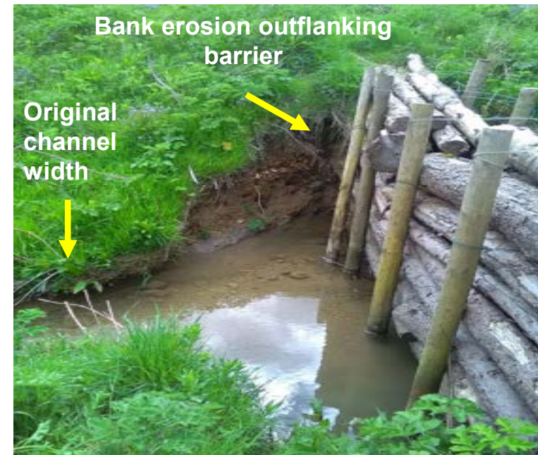
Dam which later failed catastrophically due to bank erosion
