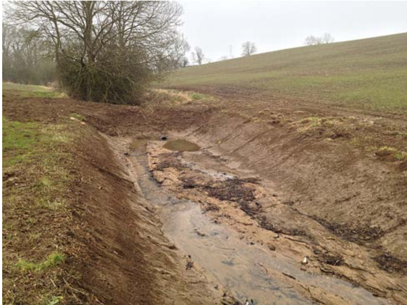
Bunded ditch on Eye Brook tributary
