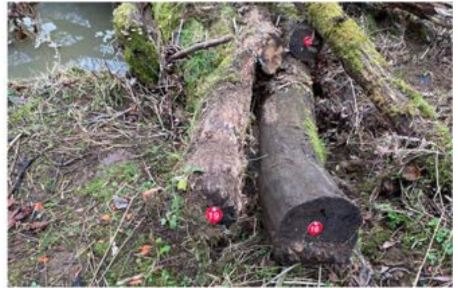
Number tags to track the logs of a degrading dam
