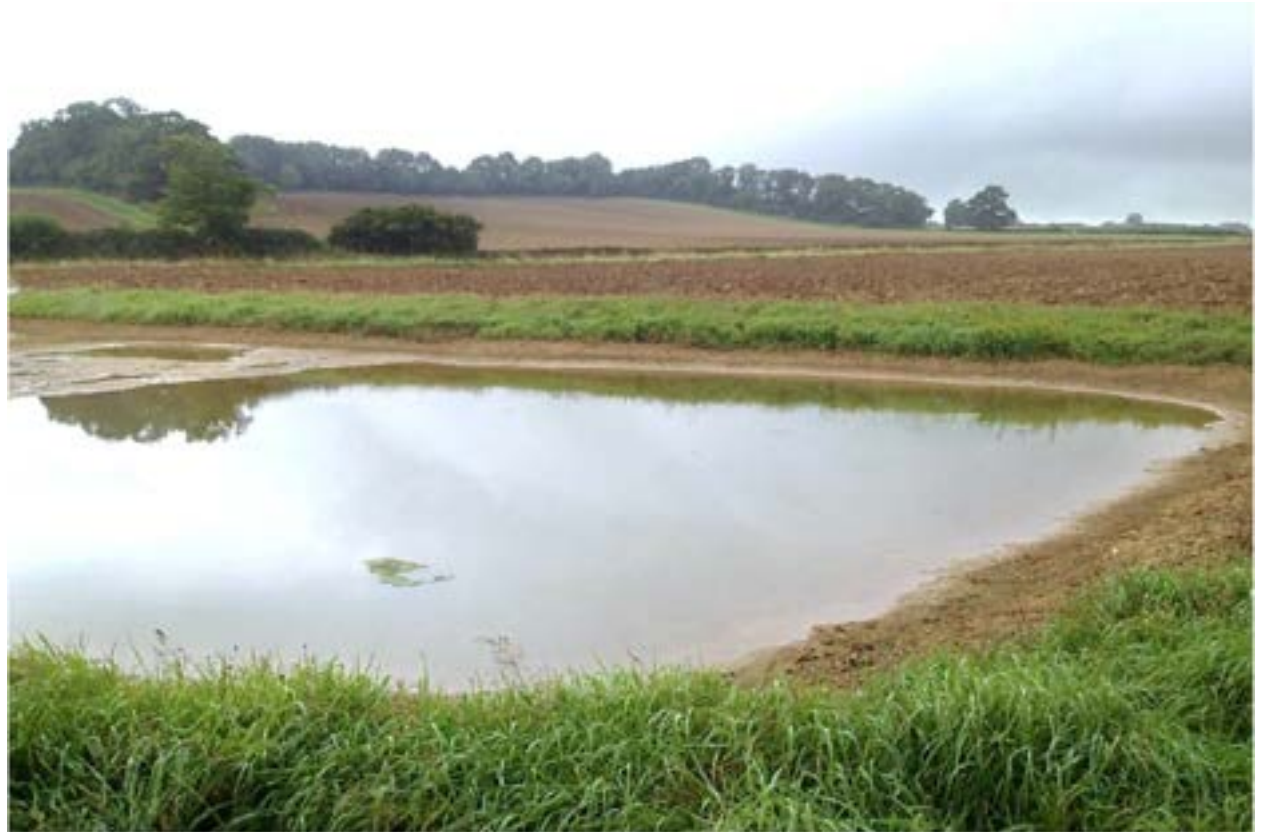
Flood storage basin on the Eye Brook
