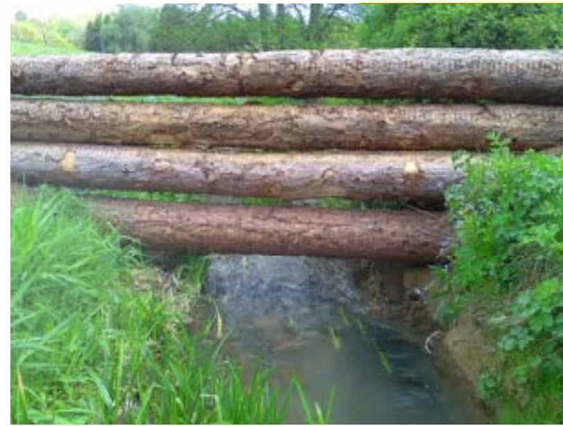
New style leaky dam on the Eye Brook
